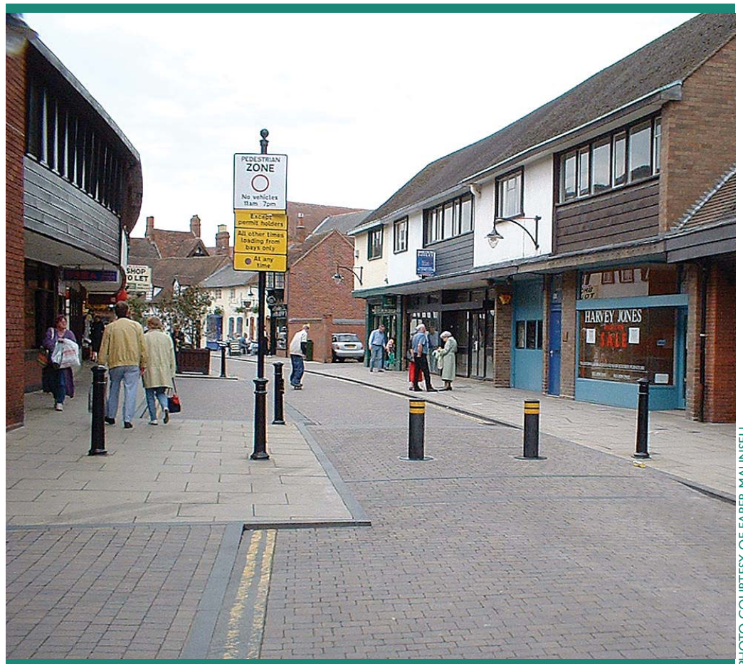
Access Control in Stratford-upon-Avon
